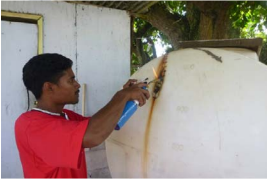
Linton fixing broken water catchment
